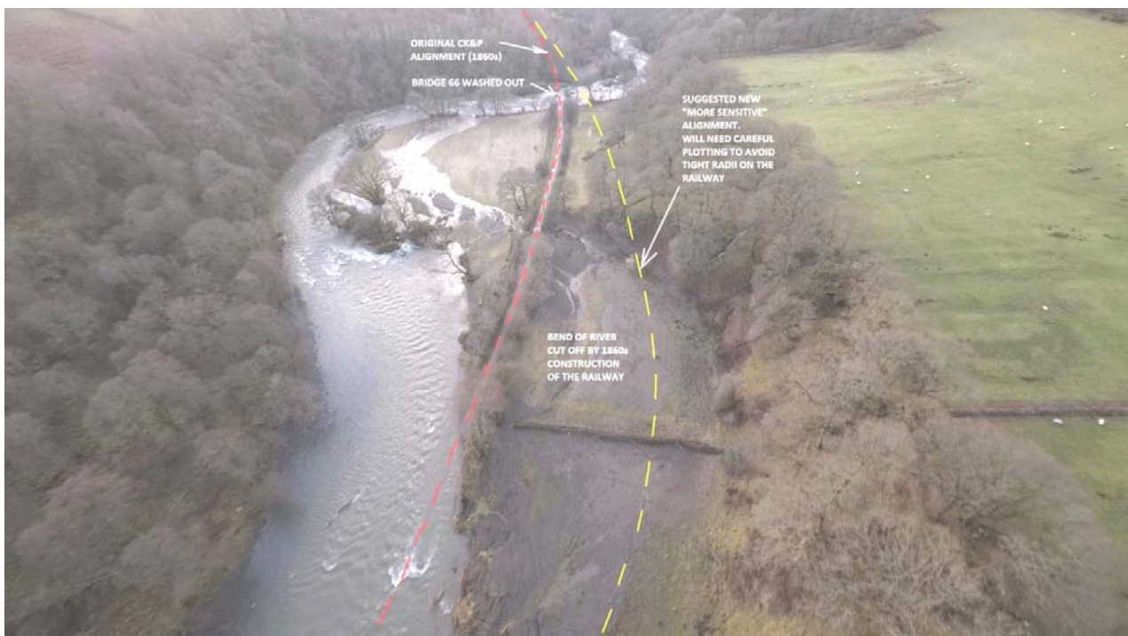
Aerial photograph (c) Terry Abraham. Annotated by Cedric Martindale
