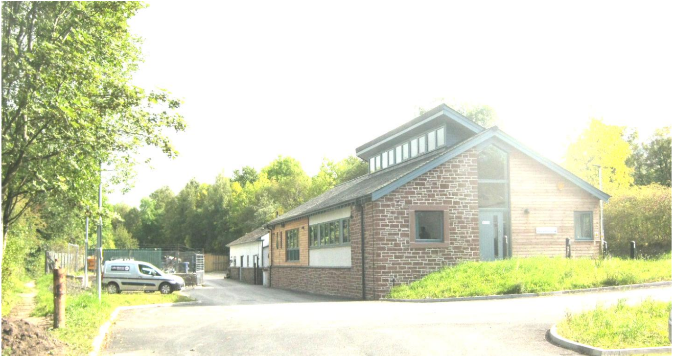
The new LDNPA facilities at Threlkeld.
