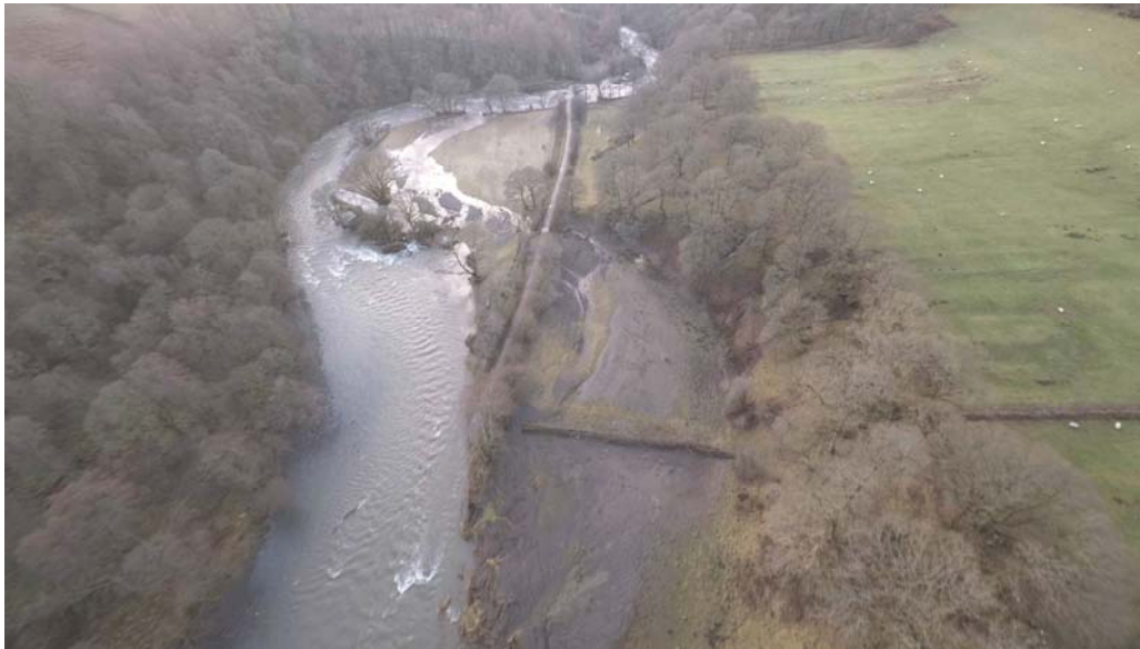
The damaged trackbed east of bridge 66 (at the top). Photograph Copyright © Terry Abraham
